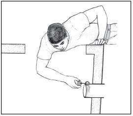
This illustration shows the gluing technique for installing a filter into a new septic tank. Installing a filter into an existing tank is a custom, site-specific job.
