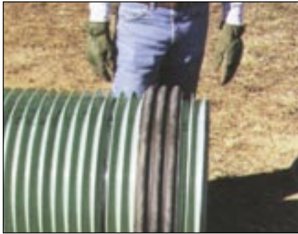
For rubber boot connections, a wide "flat top" gasket(s) is positioned under the boot to ensure a tight seal.
