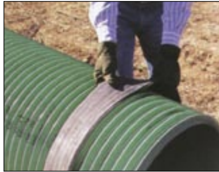
For rubber boot connections, a wide "flat top" gasket(s) is positioned under the boot to ensure a tight seal.
