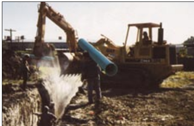
Ultra-Rib™ bears live and backfill loads, and absorbs normal on-site handling impacts without damage.
